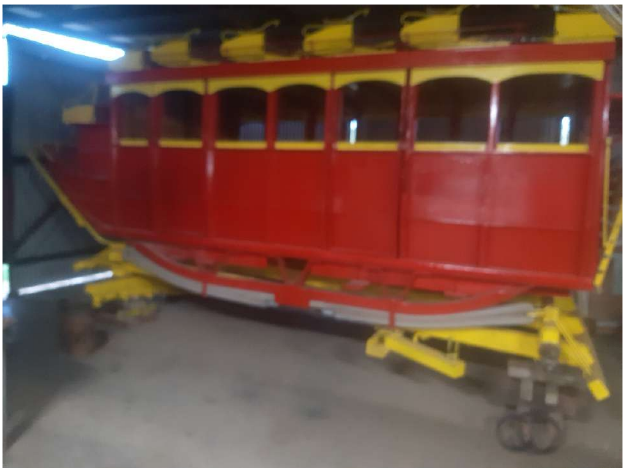
The near finished Leviathan under construction at the Teamsters Hall of Fame at Glasshouse Mountains.
