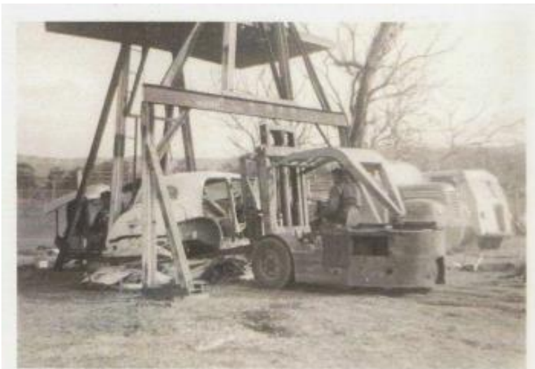
Feeding car bodies into the Crusher at Yallah.
